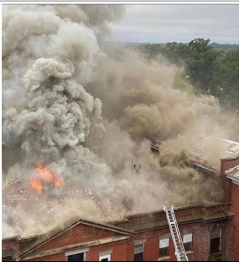
Conditions after ladder companies cut a heat hole in a common attic building fire, but just prior to the trench/ strip cut being completed.
