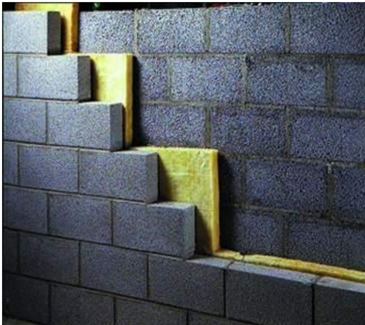
Figure 14: This wall has an inner and outer component. The inner wall is 8"x8"x16" hollow block and the outer veneer wall is 8"x4"x16" solid block. Different mortar strengths were likely used.
