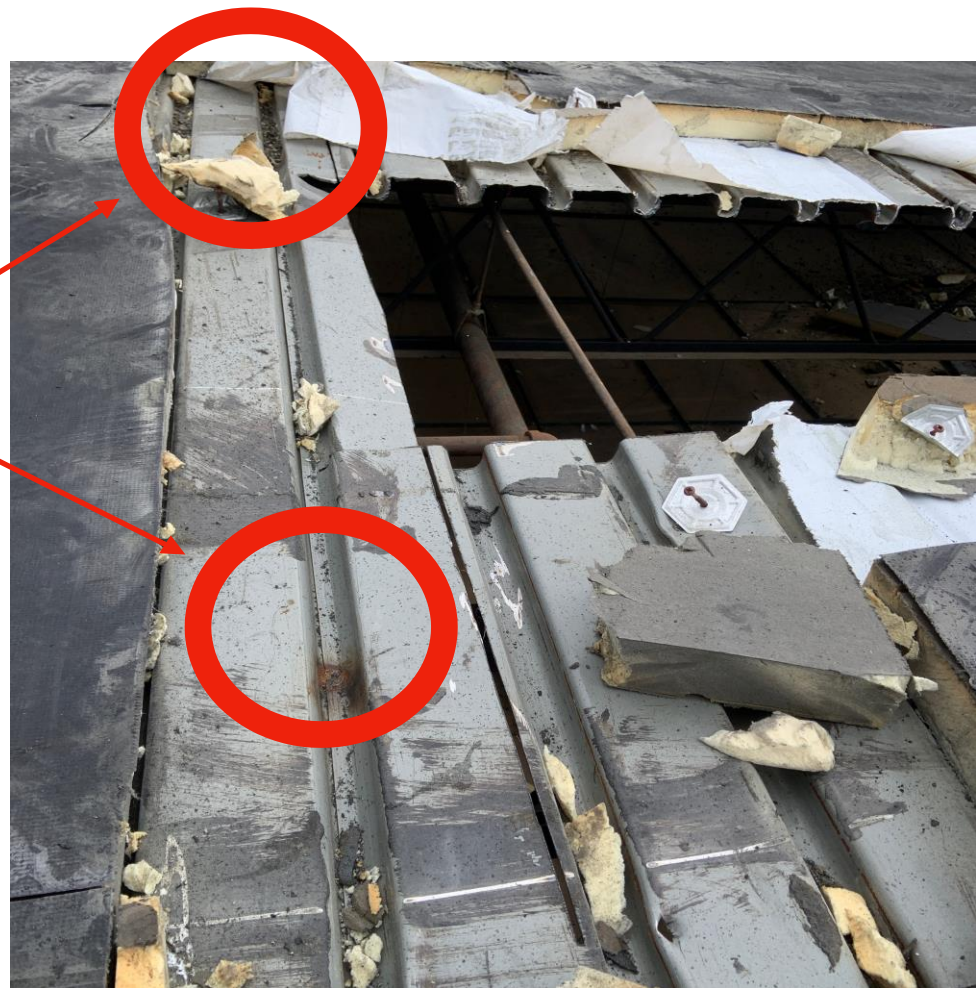
These two firefighters are running dual saws from the channel location to the end point. Due to the thickness of the decking material, a firefighter with a chainsaw has cut and already removed the initial decking to exposed just the Metal Q decking for the rotary sawyers.
