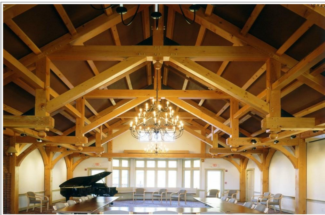
Figure 11: Once ignited, heavy timber constructed buildings present the potential for large fire volumes and rapid fire spread
