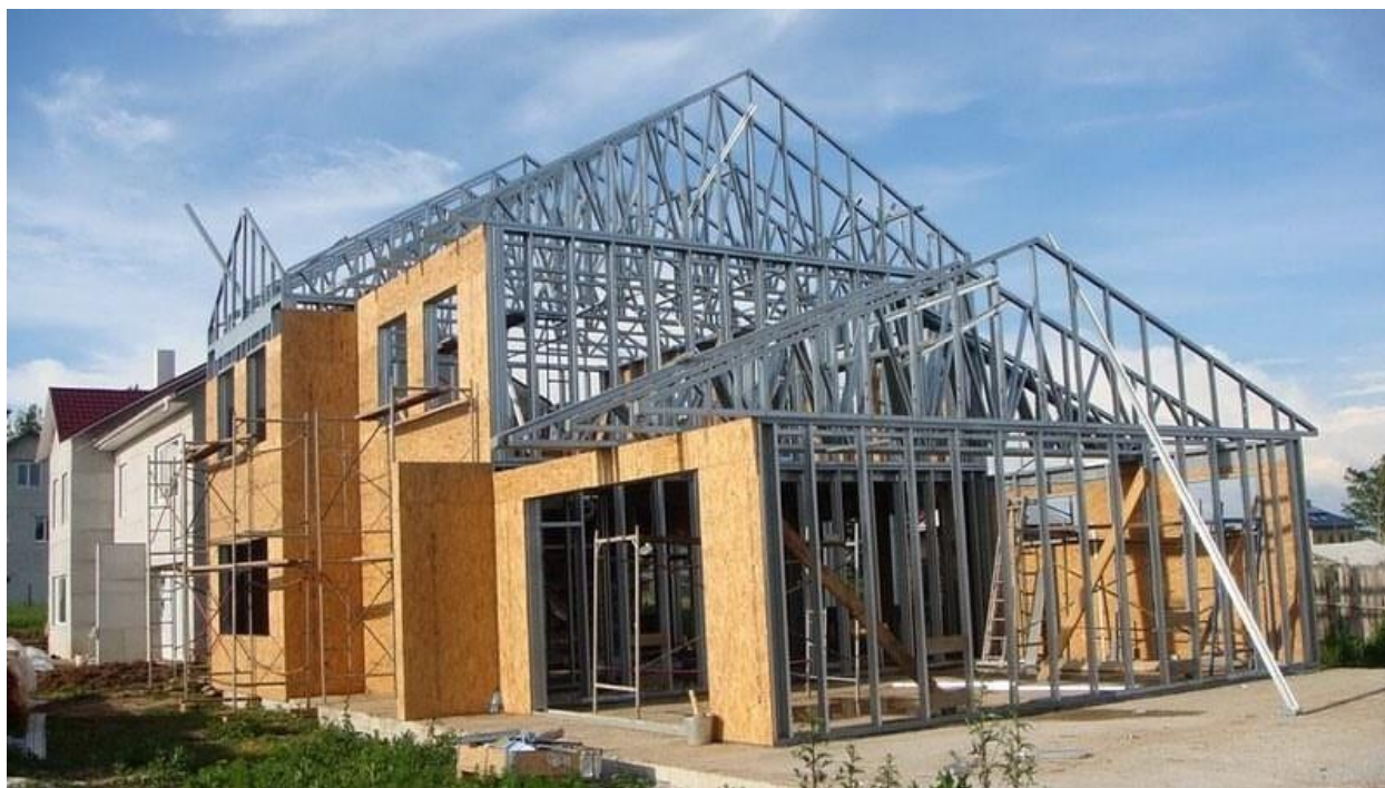
Figure 7: Steel and aluminum have become popular for framing. Commonly found in commercial applications but it is also used in residential framing.
