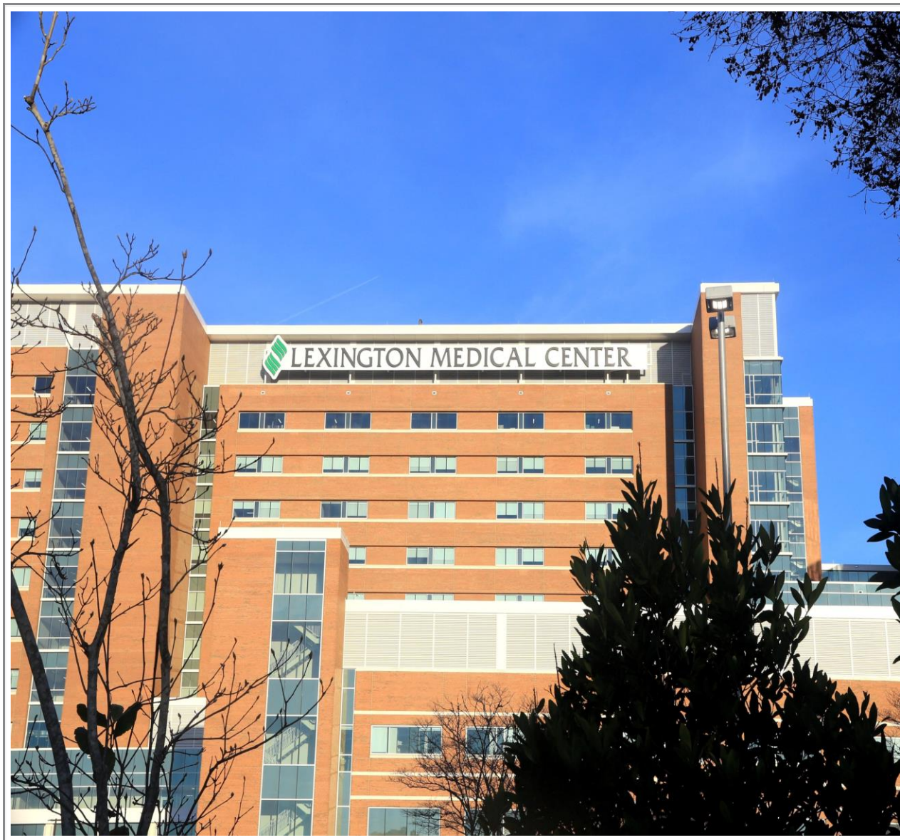
Figure 9: Lexington Medical Center Hospital is an example of a Type I building with high life hazard.
