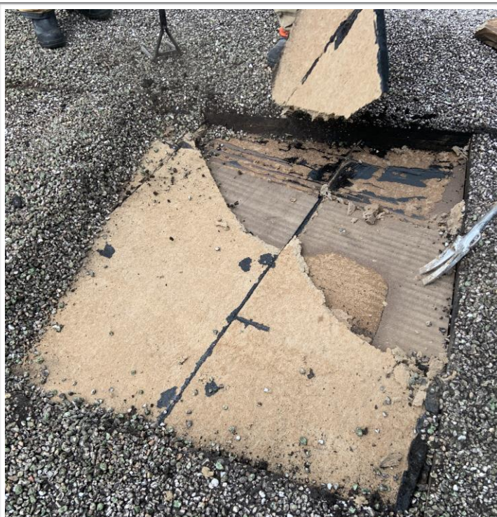
Regular fiberboard or chip lathe layering glued down.
