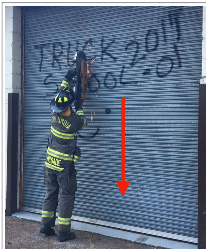
Firefighter making a single cut in the middle of this slat roll-up door.
