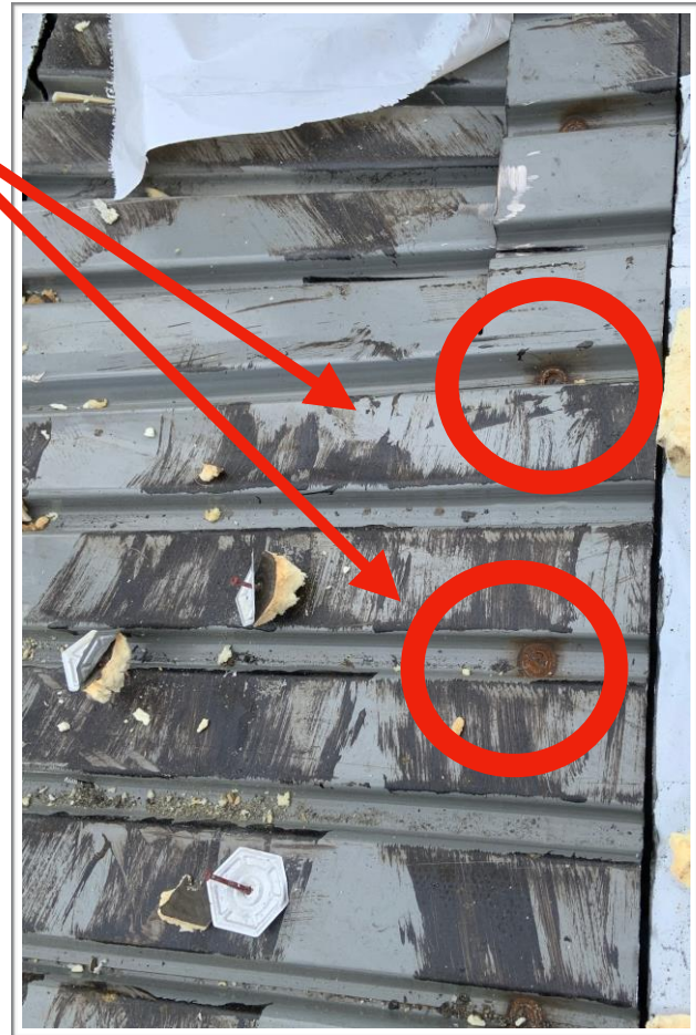
Structural Screws set into the joists
