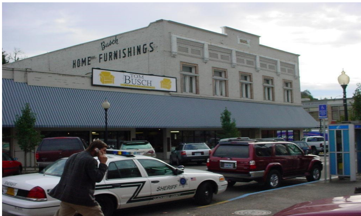
Figure 10: Buildings in a “downtown” or “Main Street” area that are type III ordinary constructed buildings.
