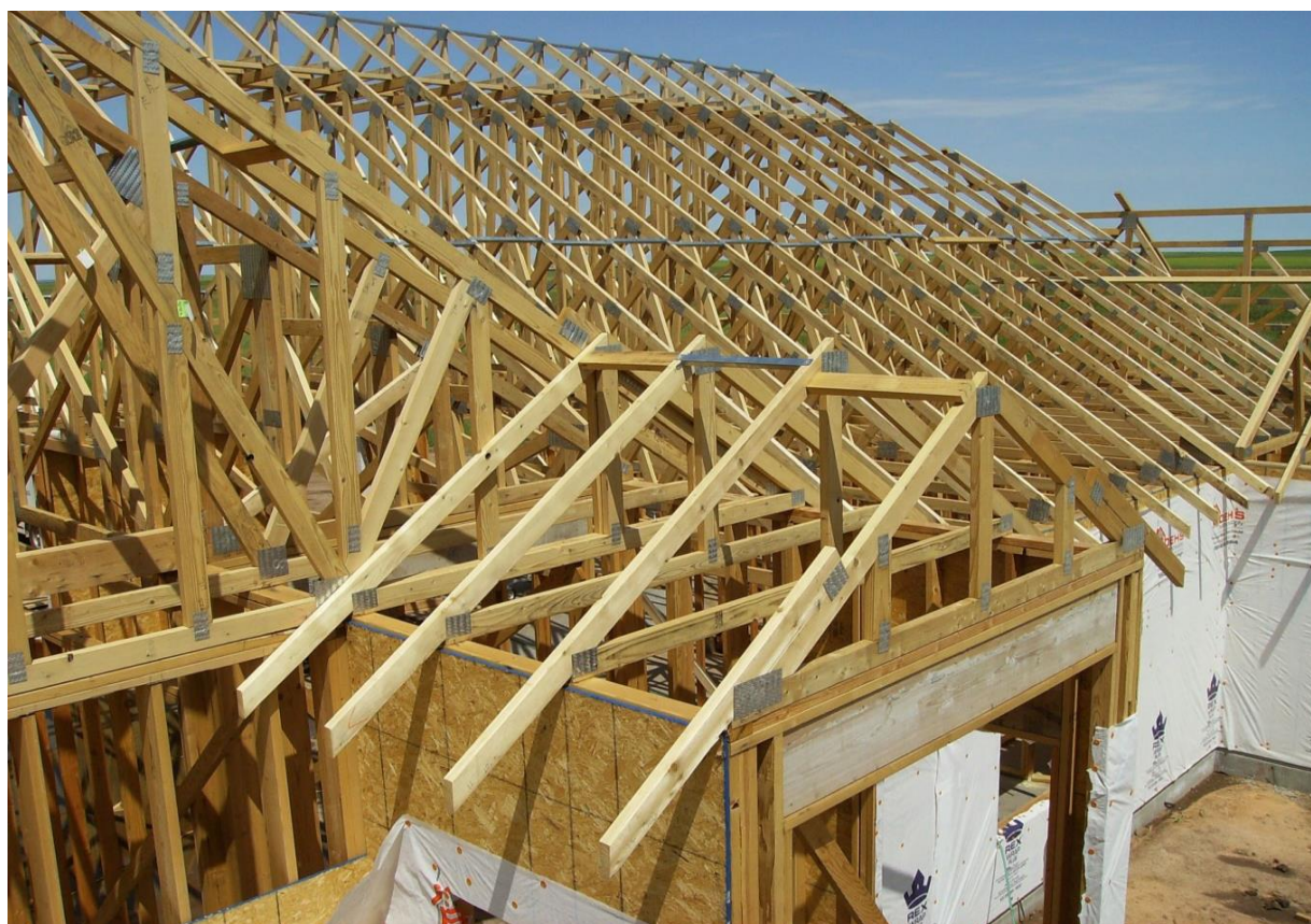
Figure 16: A common manufactured truss with metal gang plates.
