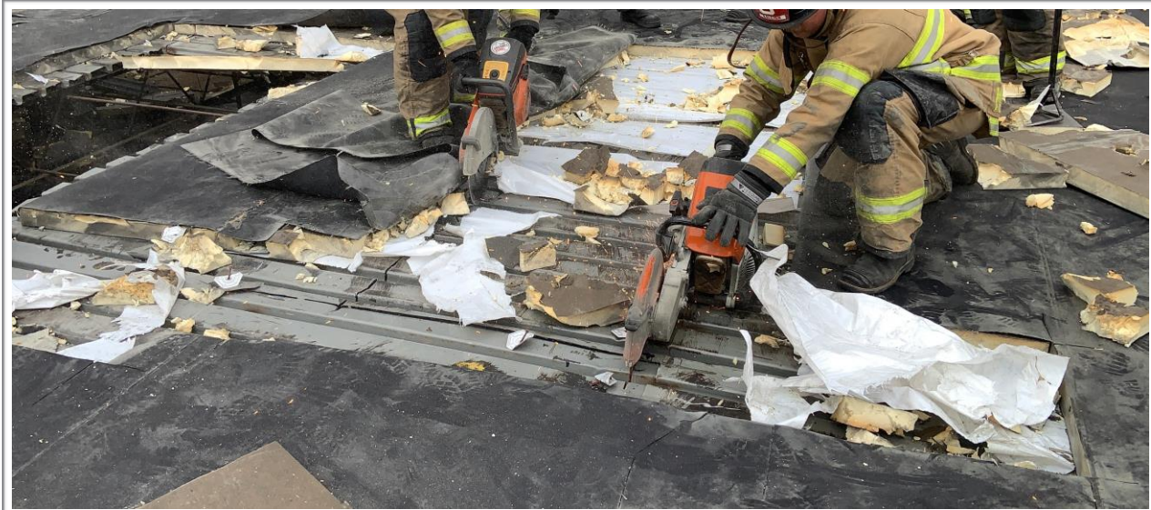
These two firefighters are running dual saws from the channel location to the end point. Due to the thickness of the decking material, a firefighter with a chainsaw has cut and already removed the initial decking to exposed just the Metal Q decking for the rotary sawyers.
