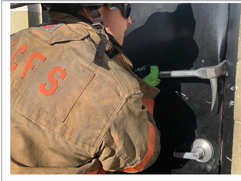
Another View of a FF using the Adz to GAP and CRUSH an outward swinging door. It is imperative to crush the door to ensure a good SET.
