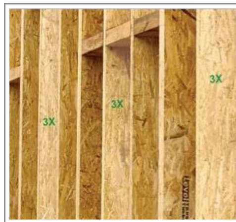
Figure 5: Timberstrand wood being used vertically
