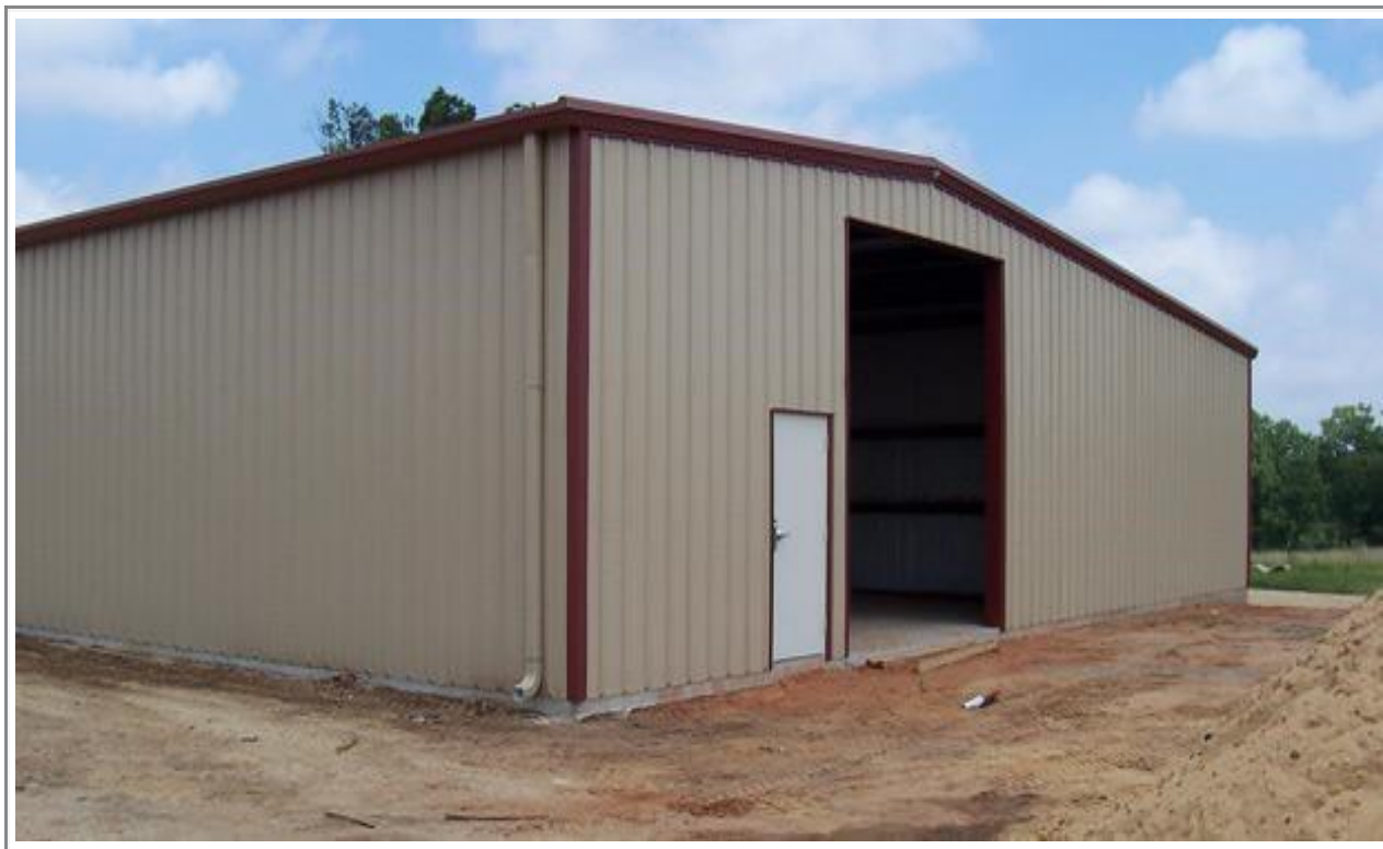
Figure 10: These types of metal clad buildings are Type IIB construction and are used for agriculture and light manufacturing. Remember, the contents and often times the roof materials are flammable.
