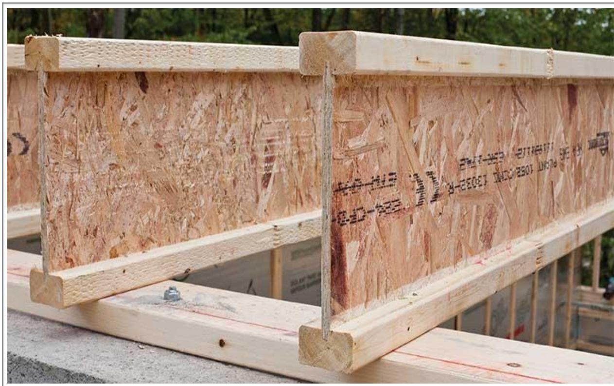
Figure 6: I-Joists being used as floor joists.
