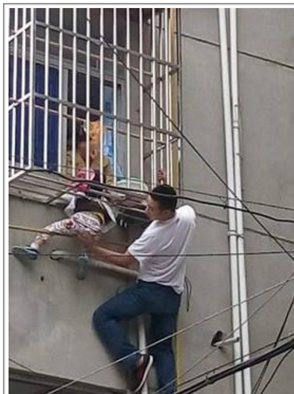
A family trying to escape a reported fire in the apartment next door, but the window gate is blocking their egress.
